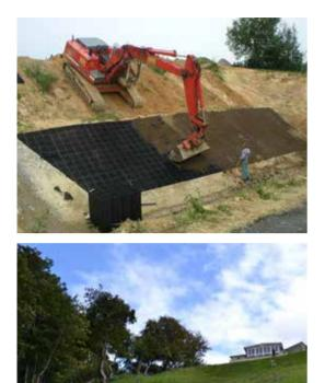
With over 200 expansion joints per square meter and 36 notched interlocking connectors per square meter the ECORASTER® counters the forces which are impacting the embankment. Erosion of the solum, soil destruction e.g. by rainwater made channels, line-shaped erosion and nutrient washout can be prevented by a proper installation of the ECORASTER® system.
