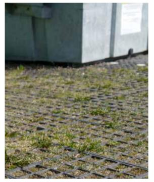
For more than 20 years, Purus Plastics has manufactured ECORASTER® permeable ground reinforcement system, made of 100% recycled materials (LDPE). Our very first installation of ECORASTER E50 "Classic" was installed over 20 years ago at a busy waste collection depot. This specific installation is found in a cold climate and the grid has been subjected to the constant freeze-thaw cycle as well as constant snow plowing.
